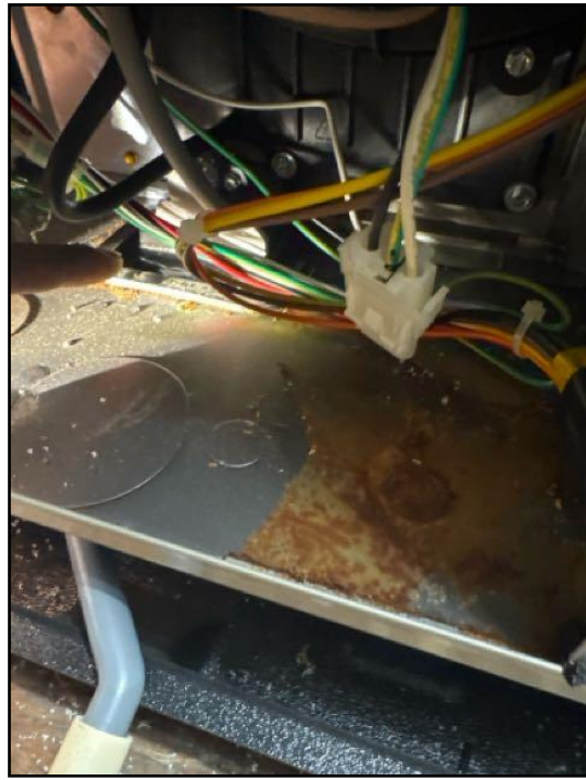
58. Condensate leak
