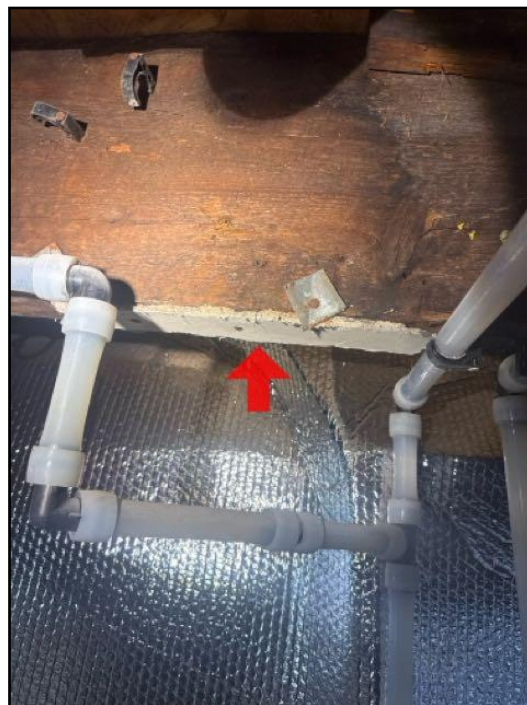
10. This includes issues such as asbestos.
