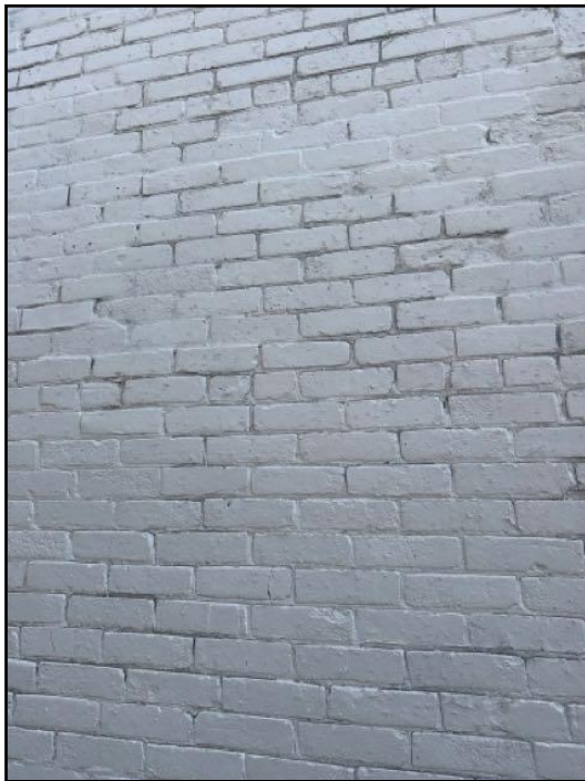
15. Mortar deterioration
