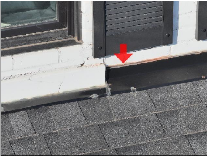
6. Not let into mortar joints
