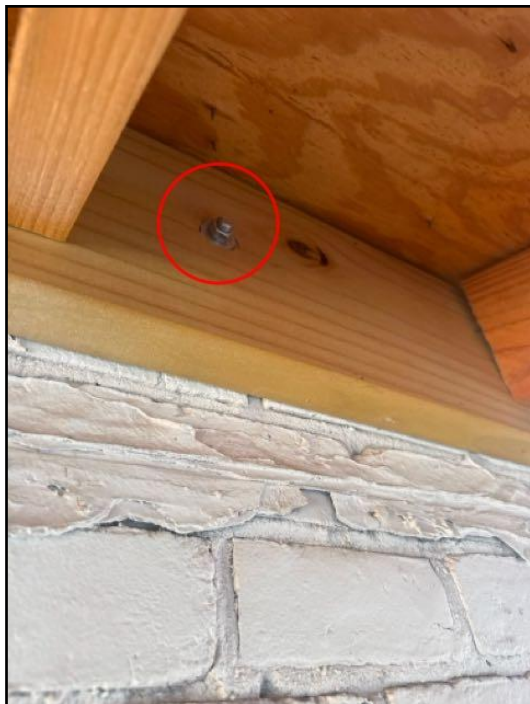
24. The front porch ledger board is fastened...
