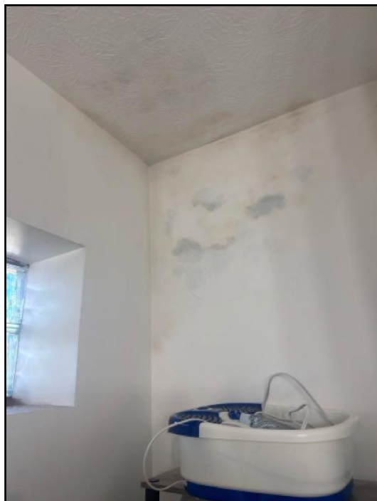
82. Water damage
