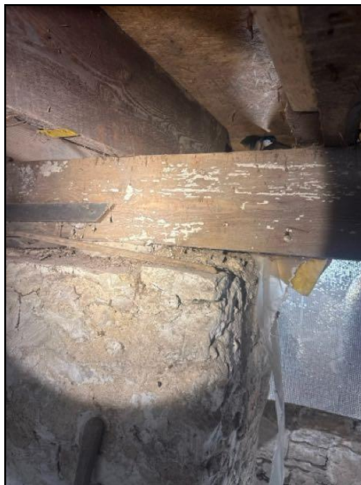
78. It has been determined that this structure...
