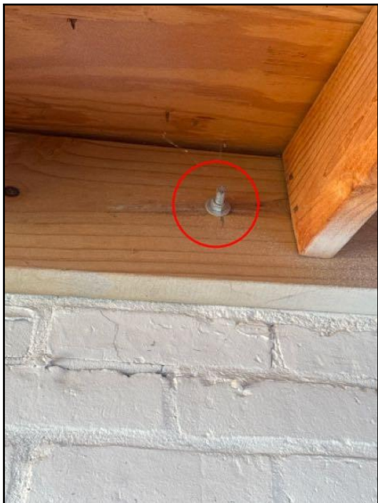
23. The front porch ledger board is fastened...
